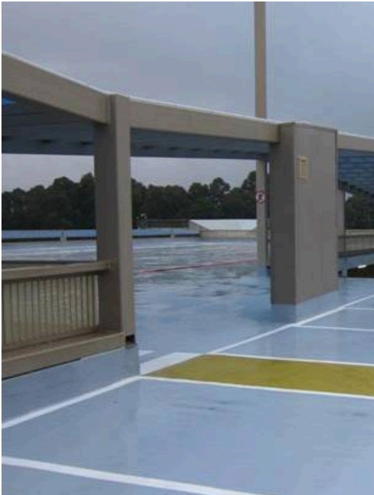
FINISH Application of TECNOTOP 2C + TECNOPLASTIC For a resistant, visually attractive and anti-slip finish.
