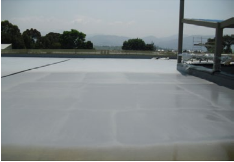
WATERPROOFING Projection of TECNOCOAT P-2049
